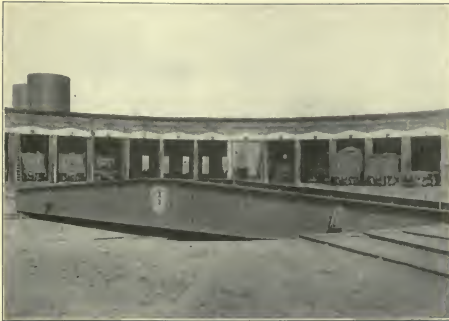
FIG. 655. FACILITIES TO BE ABANDONED. Seventy-five-foot half-through plate-girder locomotive turn-table of the Atchison, Topeka & Santa Fe Railway at the Corwith Yard engine house. This table is turned by means of an air tractor, and illustrates a type of structure which, in the event of electrification, would be rendered worthless to the railroad in its present location.
